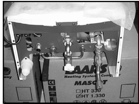
6. Assemble and tighten the following parts to make the **heating supply and cold water mains inlet** as shown below. Attach **(c)** the  $\frac{3}{4}$  copper 90° to **(l)** the red ball valve. Add **(i)** the silver 90° to **(l)**. Attach **(k)** the red handled mixing valve next. Now finish with **(e)** copper 90° and **(j)** the  $\frac{1}{2}$  copper 90°. Ensure all fittings are tight and aligned as shown.
