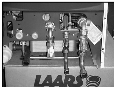
7. Connect **(j)** the ½ x 90° copper-elbow to **(h)** and tighten. Install this to **(h)** the hot water outlet.
