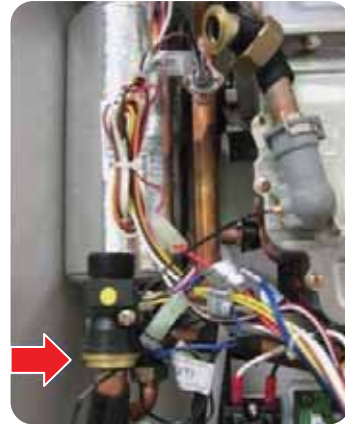
2. Remove the lower clip of the flow sensor.
