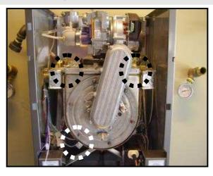
Figure 7: Upper Heat Exchanger Mounts
