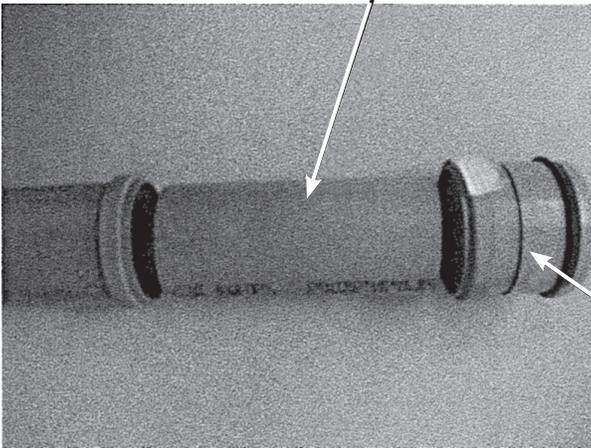
The PP to PVC adapter can either be installed on the pipe or into the vent terminal for the next step. The final step is to make sure the vent terminal is attached and secured to the adapter.
