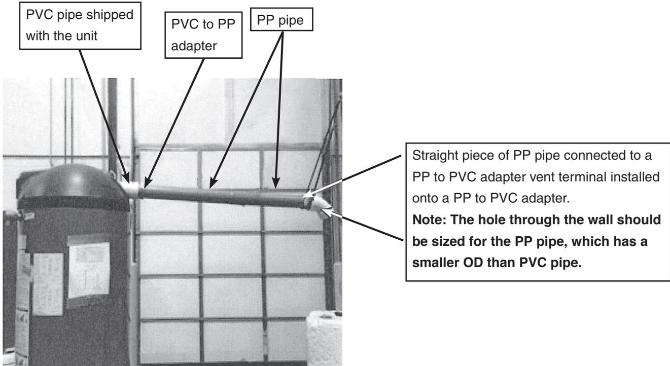
The first step to install the PP pipe is to find a PVC to PP adapter and lubricate the gasket that will slide into the PVC fitting. The lubricant for the Centrotherm parts is called Centrocerin. Apply a small amount onto your finger and then apply to the outer gasket.
