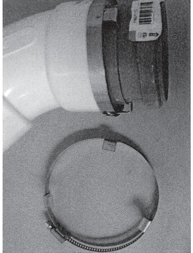
Pipe and fittings are then installed to reach the area for the vent terminations. Each bell end of the pipe has a gasket, which should be lubricated before the next piece of pipe or fitting is installed.
