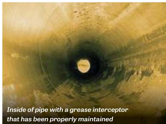
*Inside of pipe with a grease interceptor that has been properly maintained*
