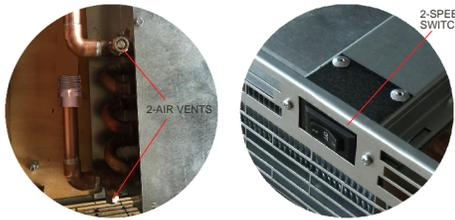
DOUBLE AIR VENT Fig. 1 SWITCH ON FRONT OF UNIT Fig. 2
