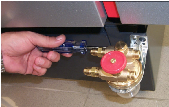
Fig. 9 Mounting filter and check valve assembly
