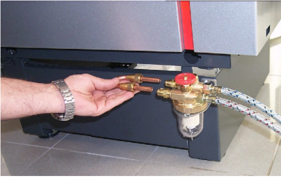
Fig. 6 Connection to a one-pipe system
